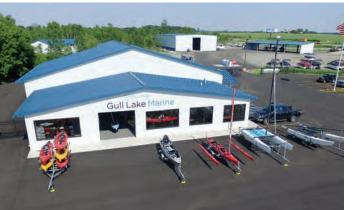
When it comes to performance, few roof systems compare to the Nucor's standing seam roof panels. Both Loc Seam-90 and Loc Seam-360 achieved a Class 90 Wind Uplift rating by Underwriters Laboratories when tested in accordance with test procedure UL 580. The Loc Seam-360 is also Factory Mutual approved and both systems have Class A fire ratings when tested in accordance with test procedures ASTM E108.
